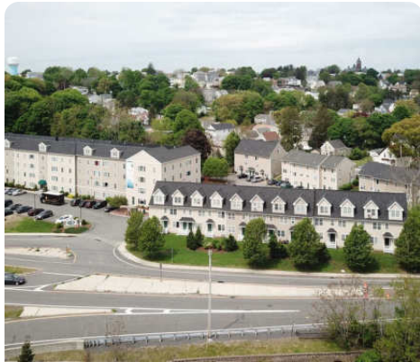
The Elora Flats & Townhomes
