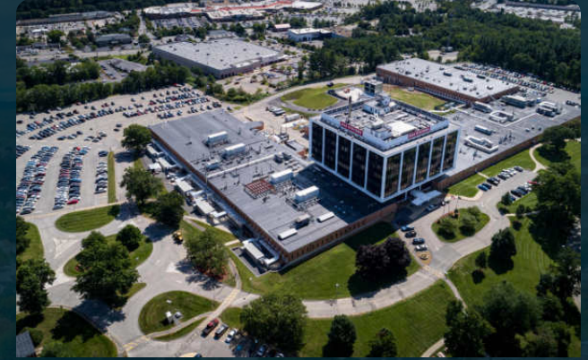
BAE Systems – Nashua Facility
