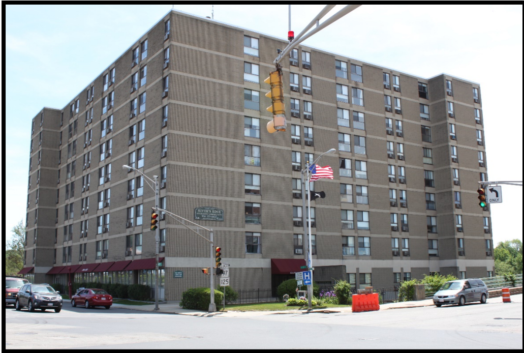
View from corner of Water and Washington
