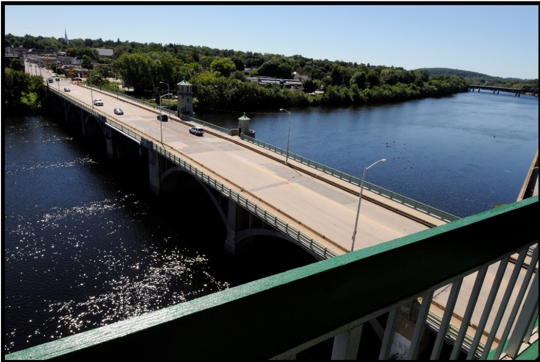
View of the Basiliere Bridge, the main overpass
