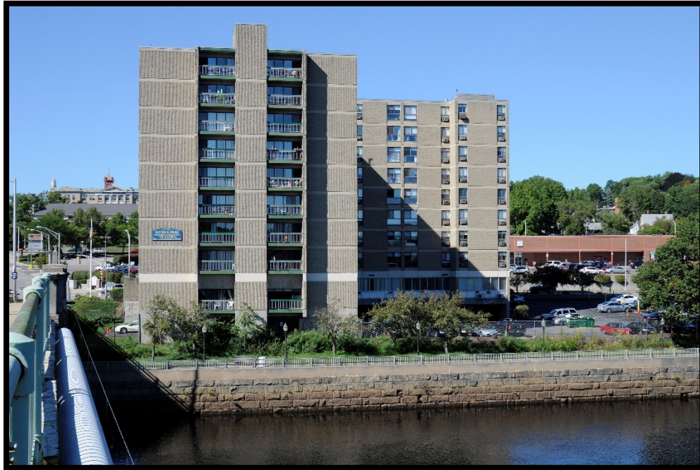
View coming over bridge entering center of Haverhill
