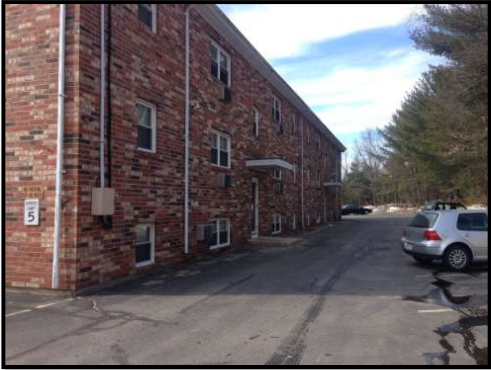
View of backside of center building and parking
