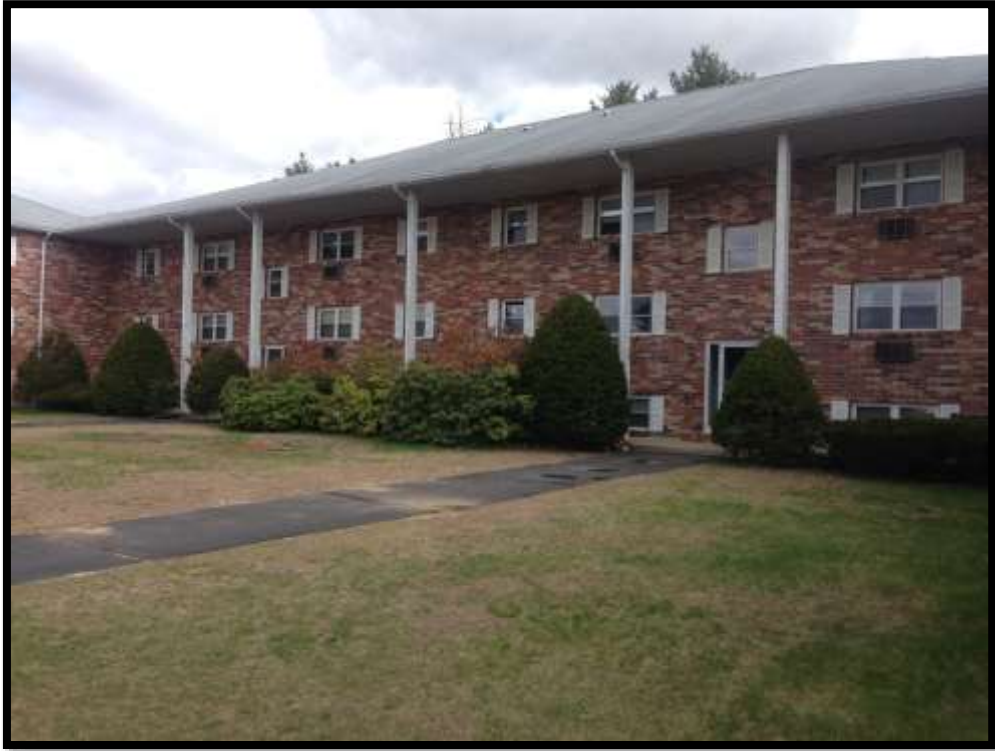
View of center building and courtyard
