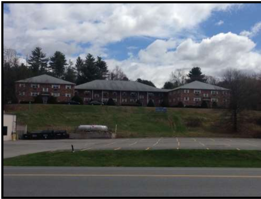
View of entire structure from route 38
