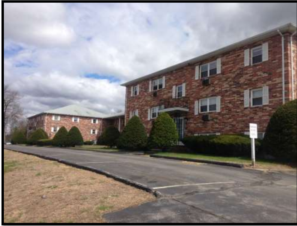
Front view from right side of driveway
