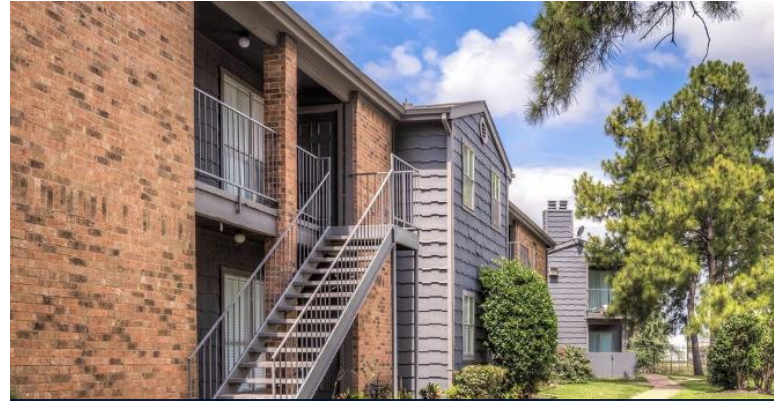
Verandas at Bear Creek 160 Units – Houston, TX
